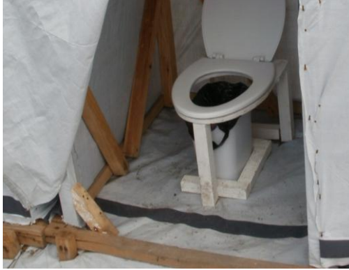
Figure 6.2 Cubicle floor & walls of plastic sheeting
