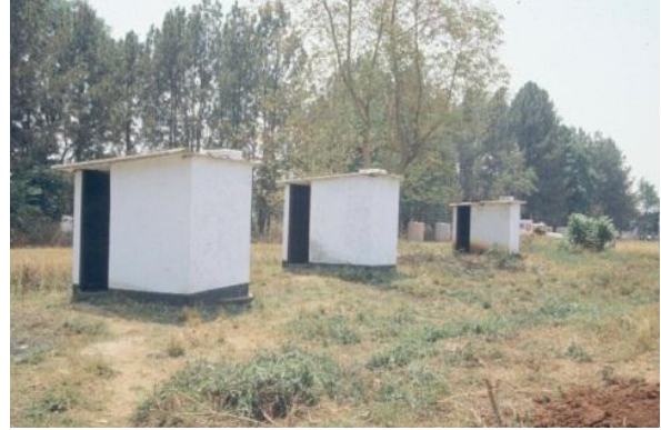
Figure 6.3 Brick cubicles on pit latrines
