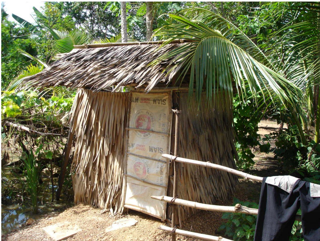
Figure 6.4 Cubicle made of palm leaf
