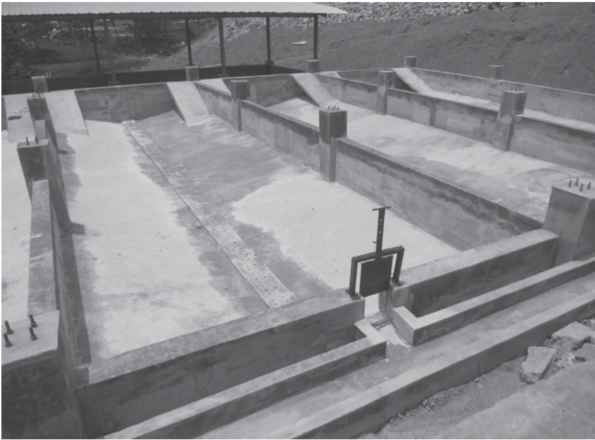
Photo 9.1 Drying beds under construction
