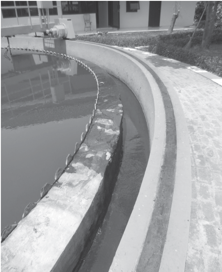
Photo 5.5 Unbalanced flow resulting from poorly levelled weir
