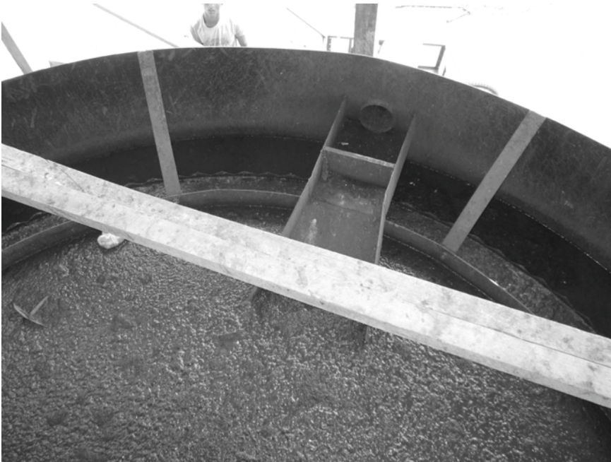
Photo 7.2 Arrangement for scum removal, Sittwe hopper-bottomed tank
