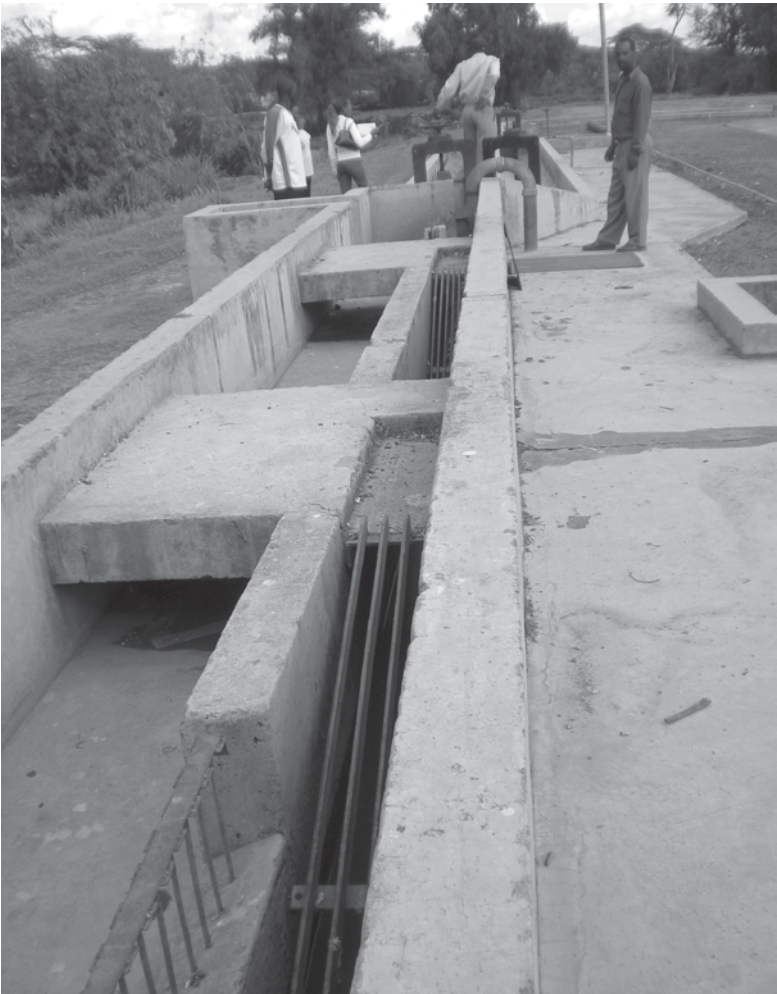
Photo 5.3 Inclined screen with operator access
