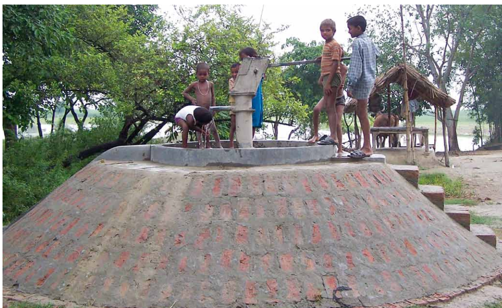
Flood-proofed Handpump in Bahraich, India: the apron is one metre high and the slope of the base gradual enough to prevent damage to the base during flash floods (Photo: District Administration, Uttar Pradesh, India).
