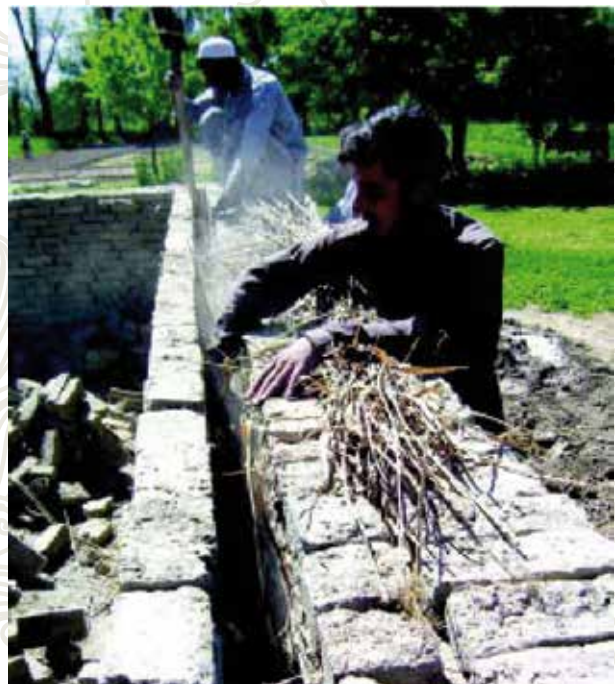
Picture No. 5: construction of the greenhouse wall – design No. 4
