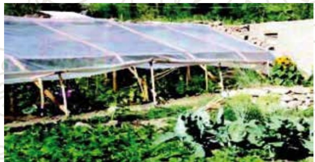
Picture No. 18: The summer ventilation of the greenhouse by lifting the bottom part of the polythene sheet.
