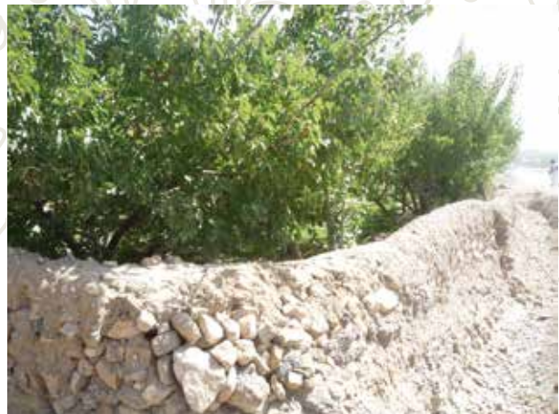
Picture No. 4: Mud walls
