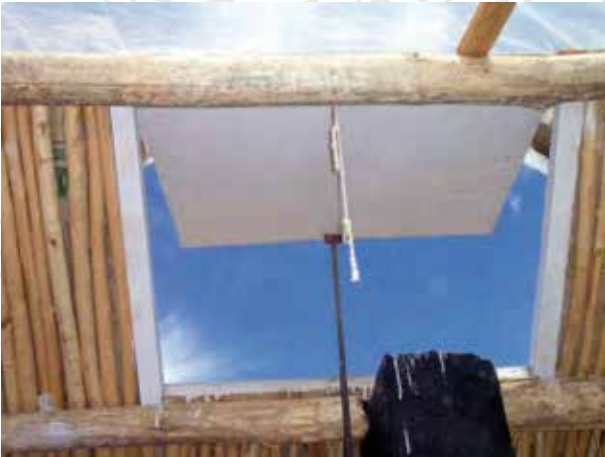
Picture No. 11: Installed and opened roof ventilator – inside view
