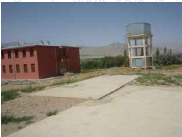
Picture No. 1: Deep well with the water reservoir; used for school and for the school field irrigation
