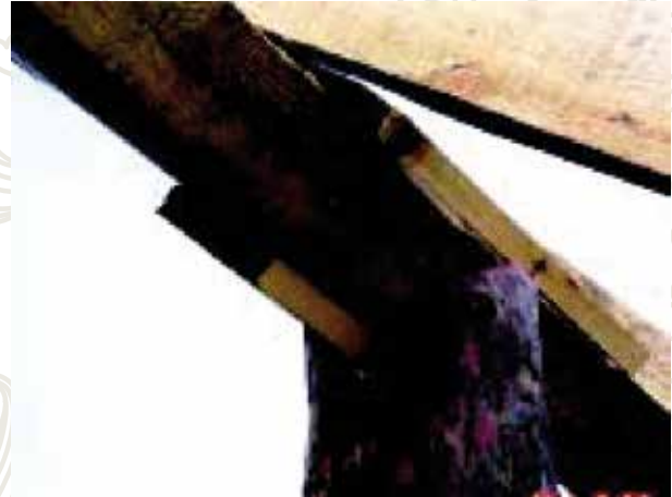
Picture No. 9: Vertical support to the jointed horizontal beams
