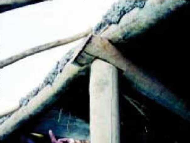
Picture No. 8: Vertical support of the main horizontal beam
