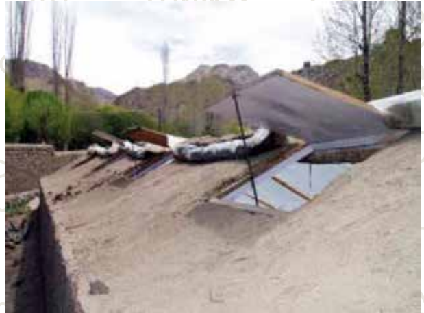
Picture No. 12: Installed and opened roof ventilators – outside view
