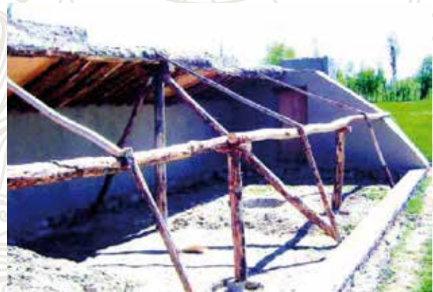
Picture No. 14: Adjusted skeleton for fixation of the polythene sheet
